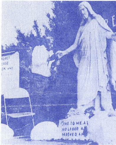
Prince George Hardison repairs hand on statue of Christ at Waterbury Holy Land.
